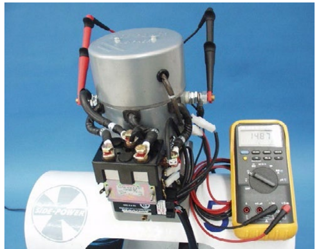
Checking voltage at thruster
