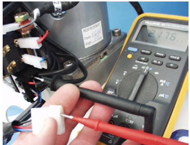
Checking continuity between black in motor pigtail and control box plug
